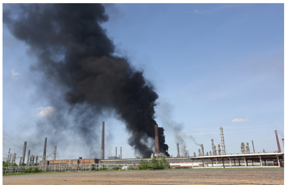
Shell Refinery Wesseling
